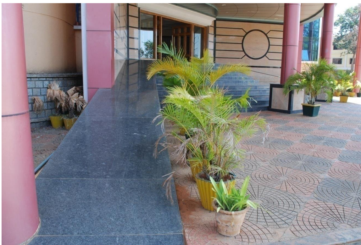
Ramp facility for disabled
